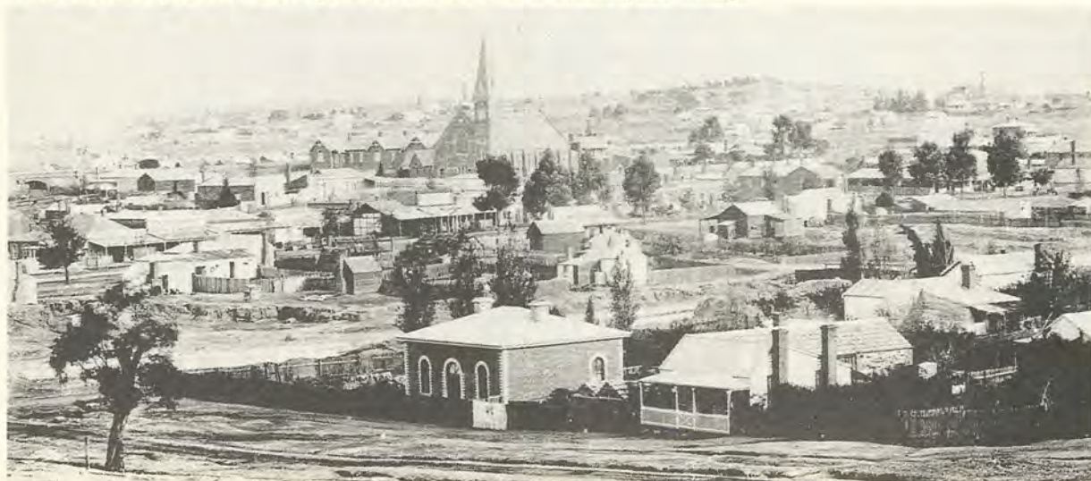
A cathedral amongst the miners' cottages: the Methodist Church at Golden Square, Bendigo.
